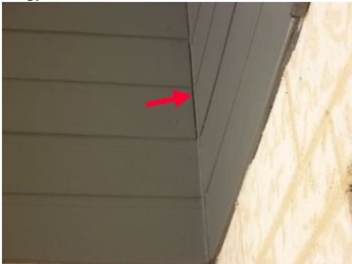
Gaps in Cladding Joints
