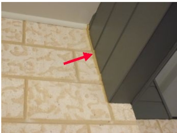
Different Colour Mortar
