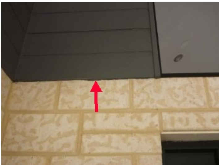
Paint on Brickwork
