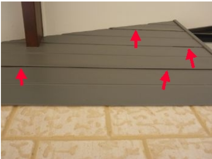
Gaps in Cladding Joints
