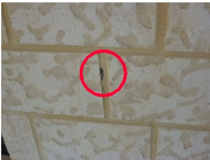
Paint on Brickwork
