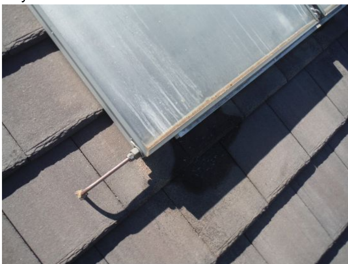
Noted small moisture stain, monitor this are. May be condensation.
