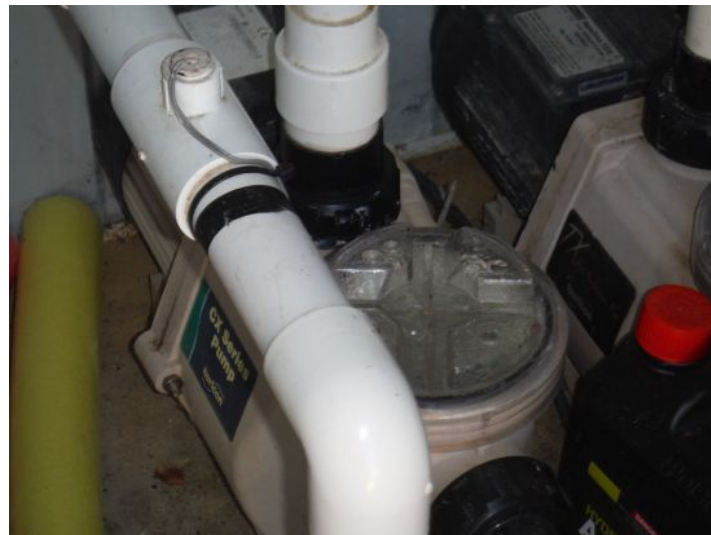
Not tested in our inspection.
