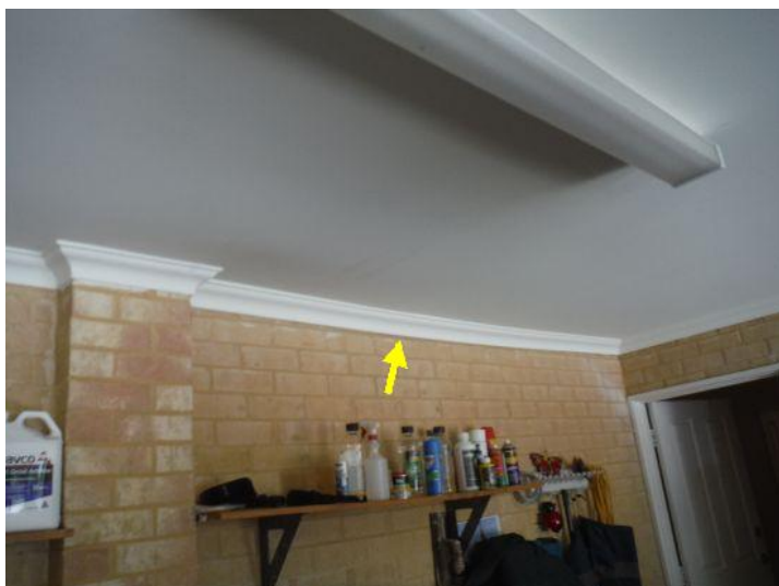
Slight sagging noted in the garage. Monitor for maintenance.
