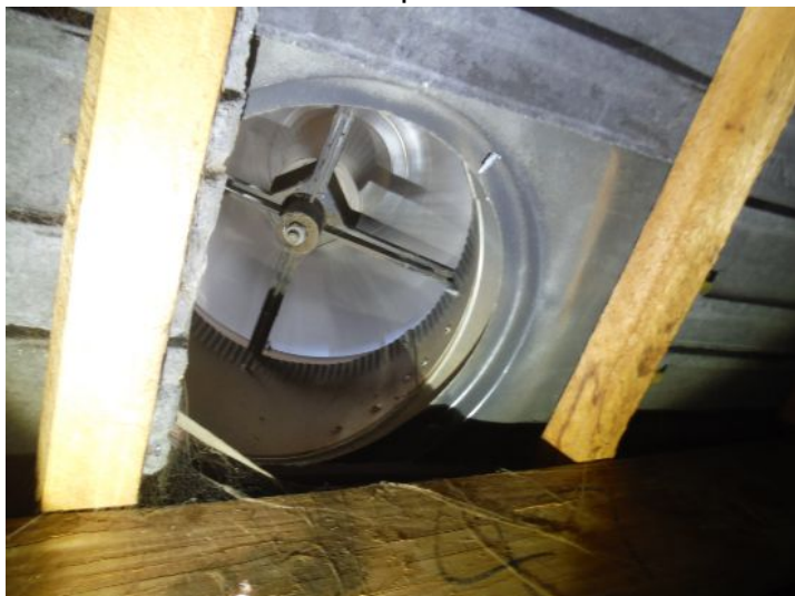
Noted the rood ventilation fan is very noisy. Recommend maintenance or replacement.
