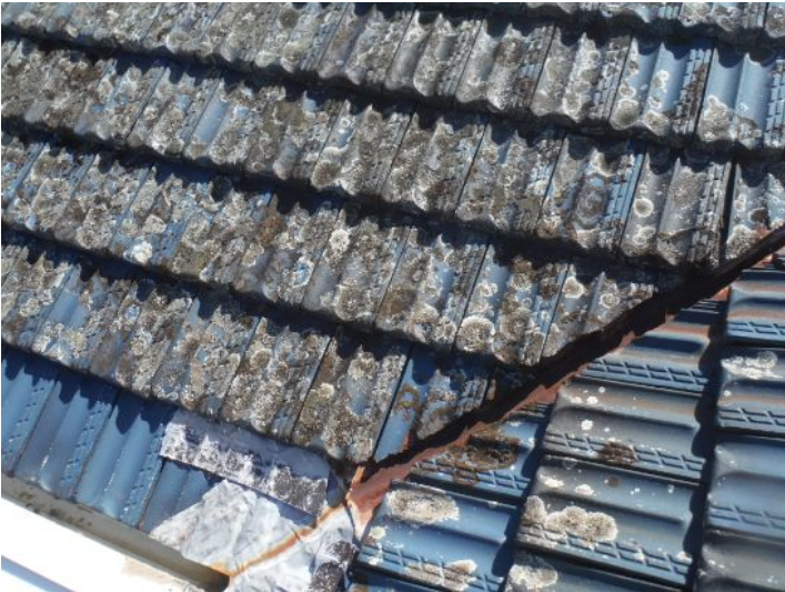
Corroded flashing noted
