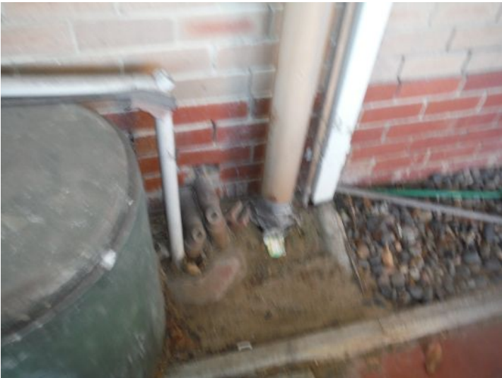
Corroded vent pipe noted.
