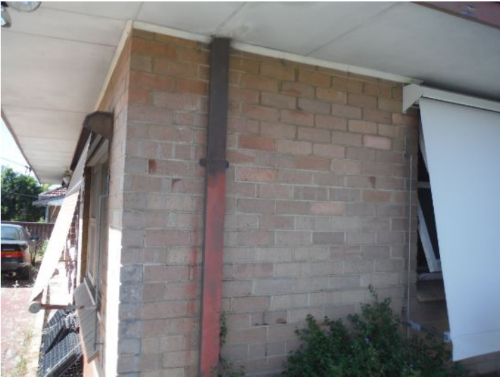
Corroded vent pipe noted.
