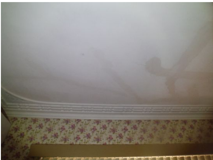
Some surface cracks have been filled in the past at the front bedroom ceiling
