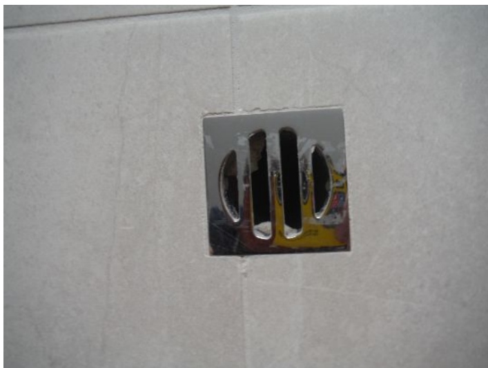
Grout in the floor grates and drain pipe to clear.
