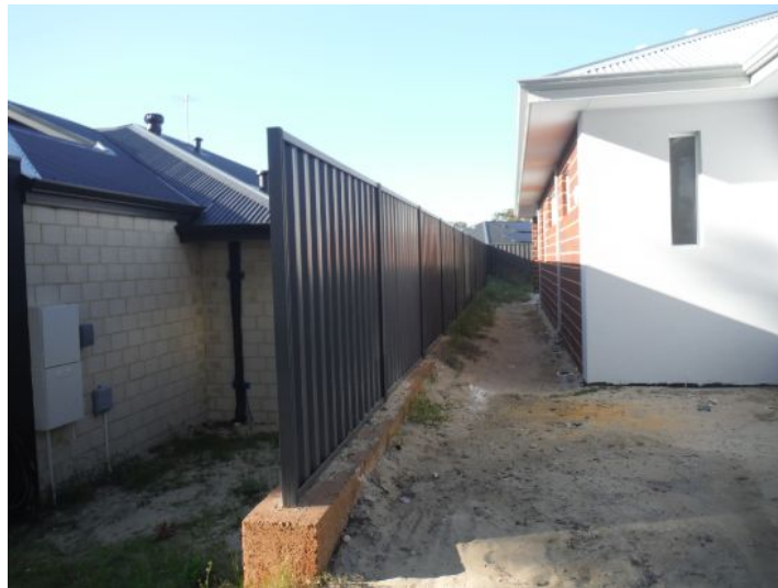
No side gate present.
