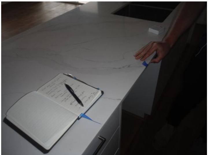
Some silicone to clean off the work top and edges.
