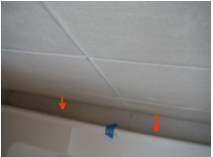
The end of the bath need the grout and sealer cleaned off
