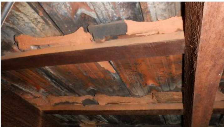
Noted some tile edges have flaked in areas, monitor for maintenance
