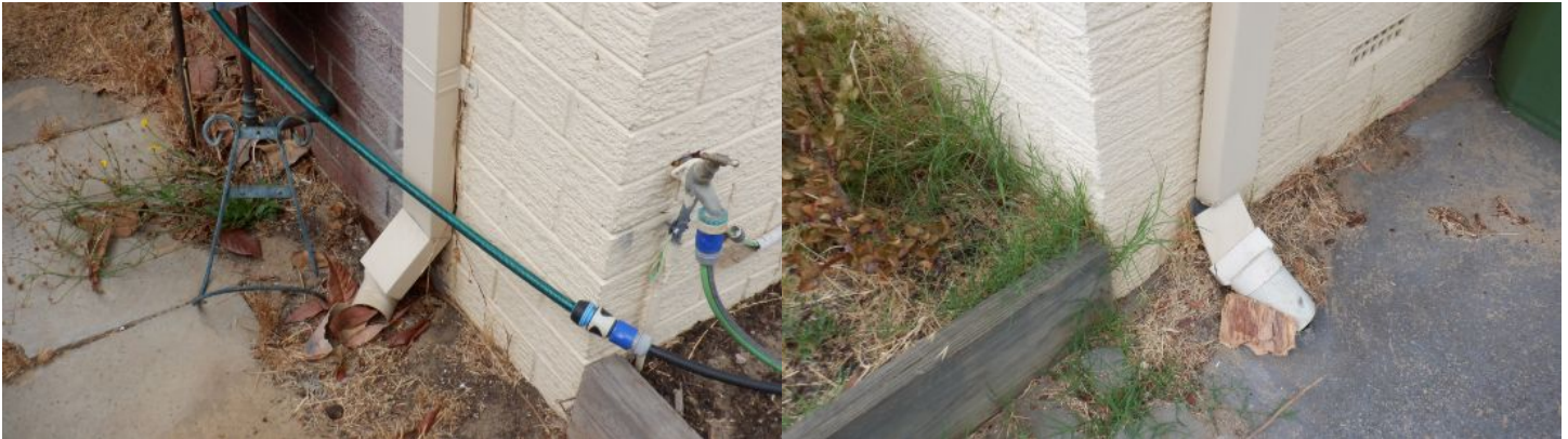
Noted broken connector, maintenance
