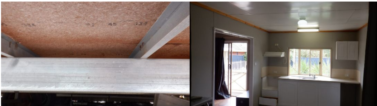
Granny flat floor structure
