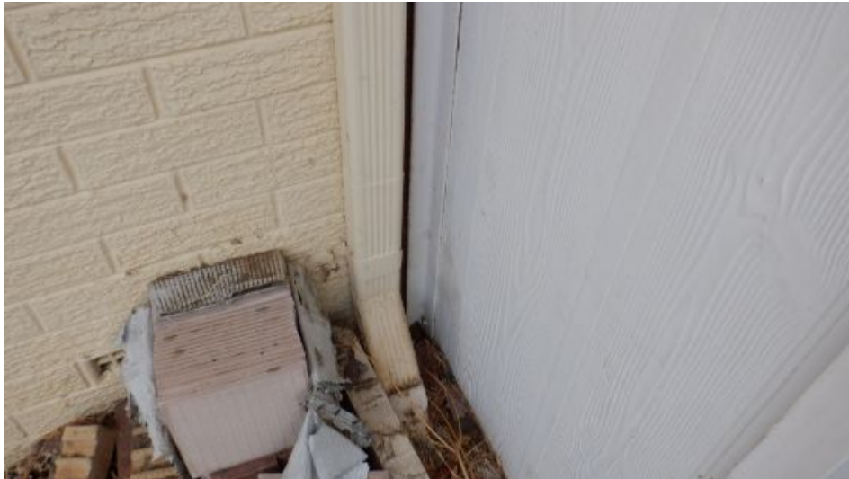
Noted broken connector, maintenance
