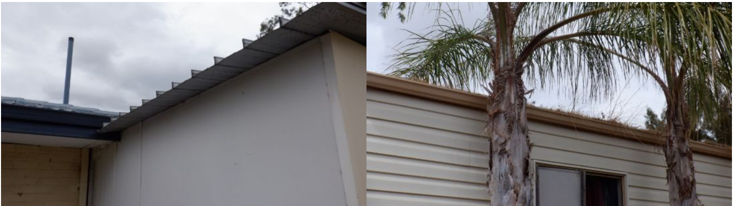
Side extension has no guttering fitted
