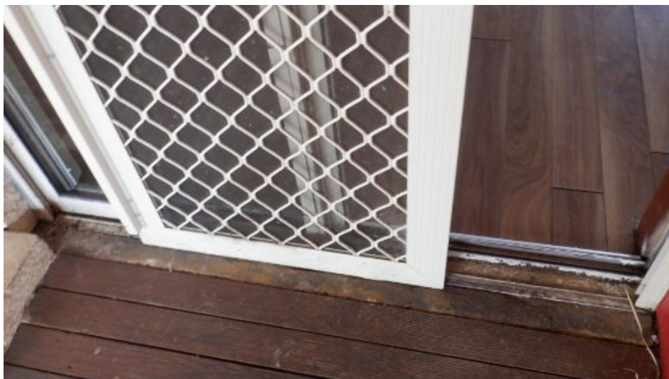
The rear fly screen door needs refitting on the track / servicing
