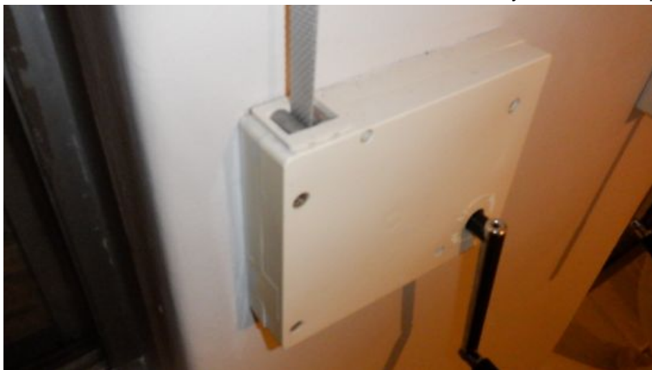
One front bedroom shutter winder requires maintenance to operate
