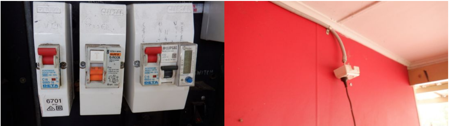
The external wall outlet needs re fixing
