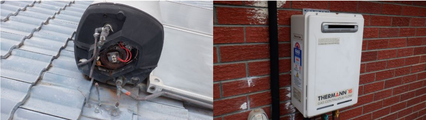
Disconnected solar tank and panels are present on the roof
