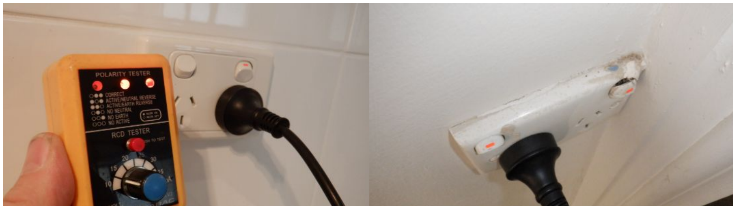
Noted loose rocker switch, side extension.
