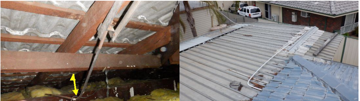
Noted steel support brace is missing
