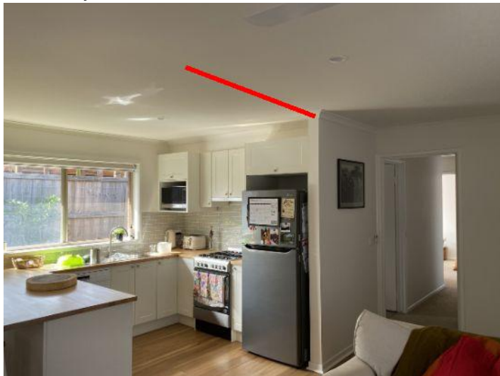
Red line indicates where the internal wall was originally located
